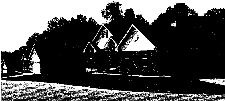
The Bailey Subdivision began constructing homes about two years ago. This NID project will result in 272 new homes in Festus.
