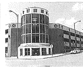
Downtown Parking Garage City of Columbia, MO
